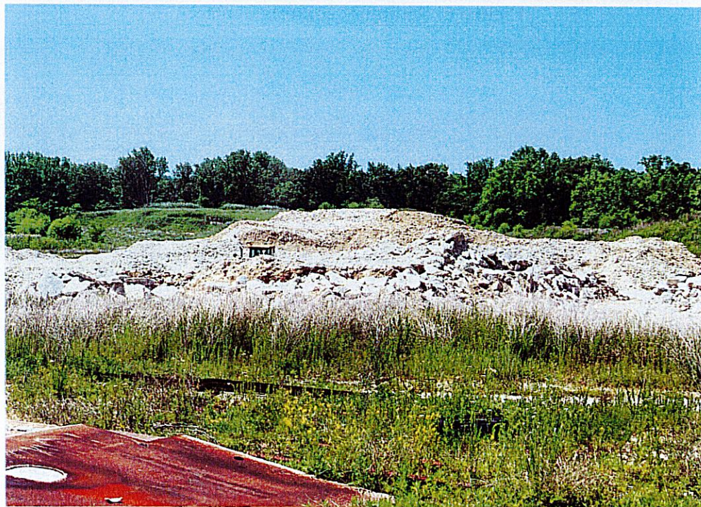
Figure 5: Reclamation underway to the Southwest
