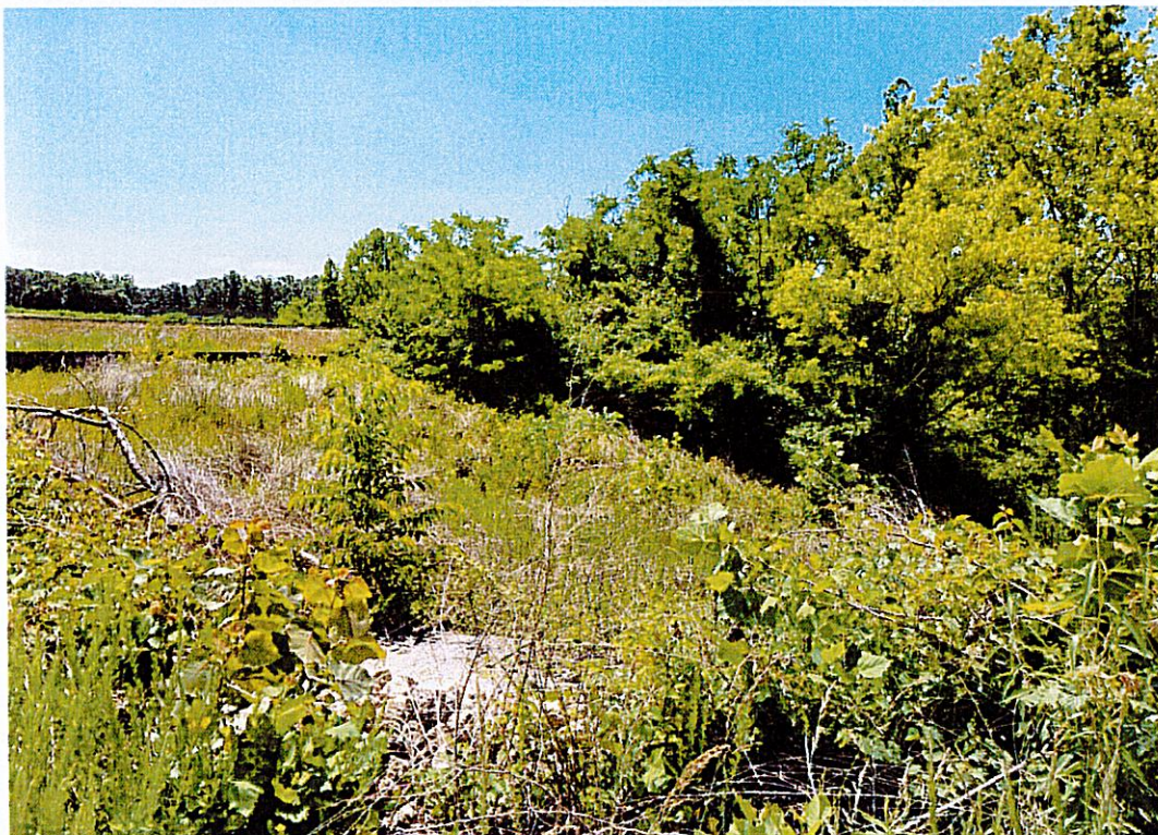
Figure 6: Sediment controls in place
