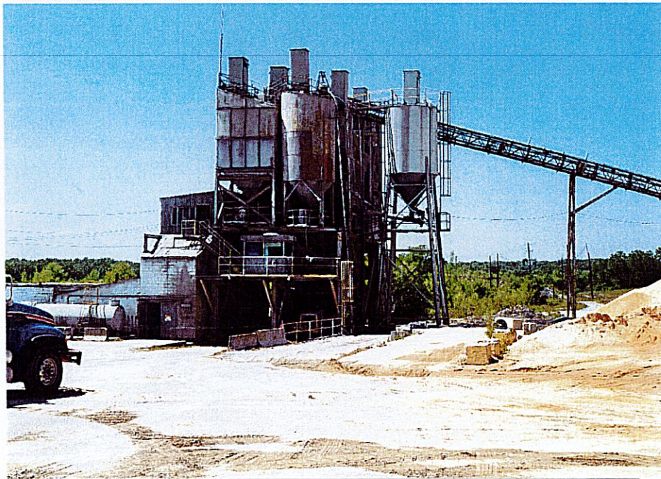
Figure 3: Active concrete plant
