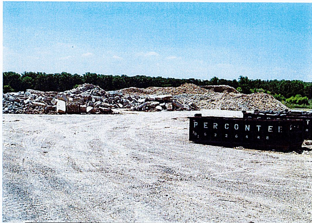
Figure 4: Stockpiled material west of plant
